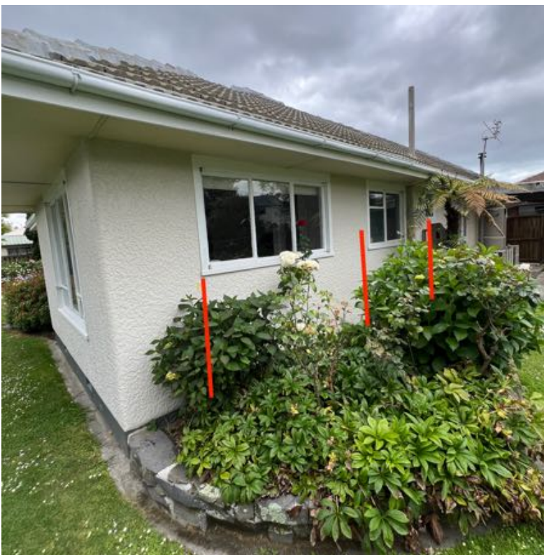
Figure 9 & 10: South elevation. Signs of cracking in Stucco.
